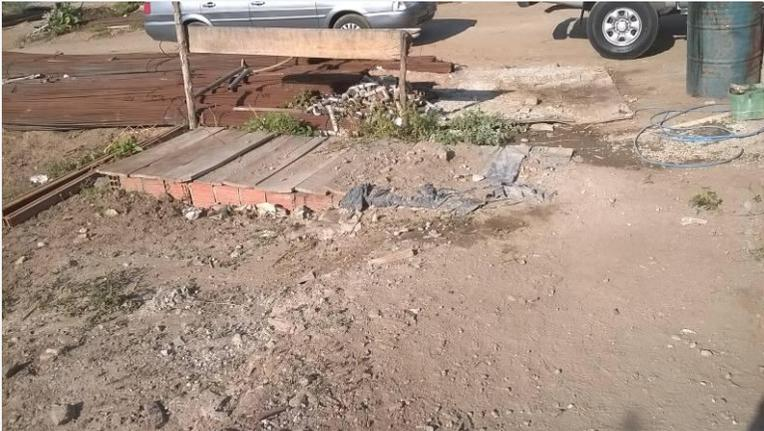
A photograph showing a makeshift septic pit. The pit is lined with wooden planks and is situated in a dirt area. In the background, there is a silver car and a blue barrel.                    |
